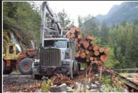
The logs are hauled to water, and then, as a bundle, pushed into the water.
