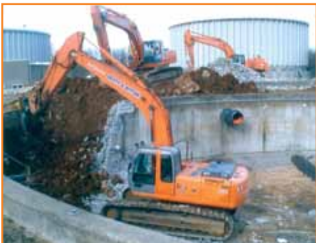
Three Hitachi excavators work a job for Bowling Green Municipal Utilities.
