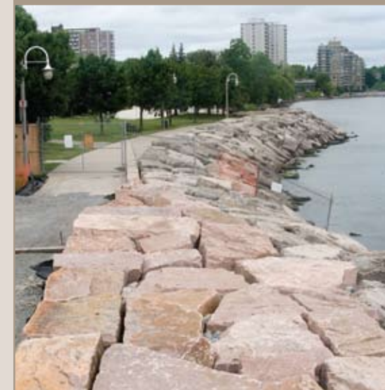
At the Brant Street Pier, an area that is prone to high winds and waves, an EX450 placed massive boulders for erosion control. Rocks often exceeded eight tons, and had to be strategically placed for the best fit.
